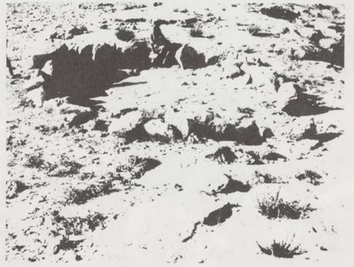
416. Circular foundation of conical stone house in the Negev, dating to the beginning of the second millennium B.C. (see page 77-81 on)
